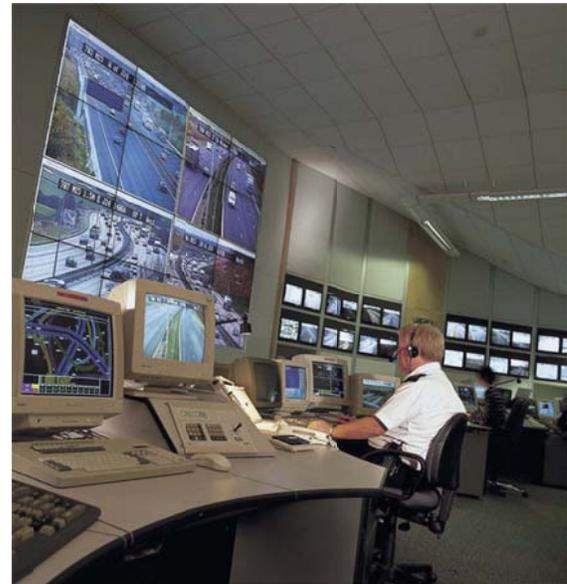
Figure 4: Inside a traffic command centre - video cameras are used in most major cities (after [6, 8])
